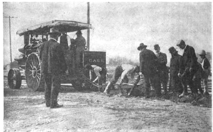
Breaking Ground for Road Improvement Outside Detroit.
